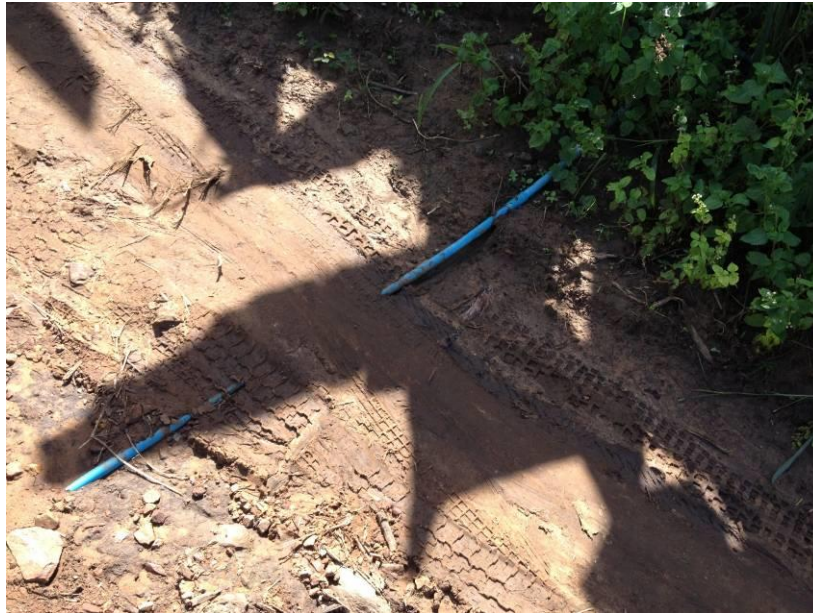
Figure 17: Water distribution system pipe in village. Pipes may be covered or above ground in the village due to mudslides.
