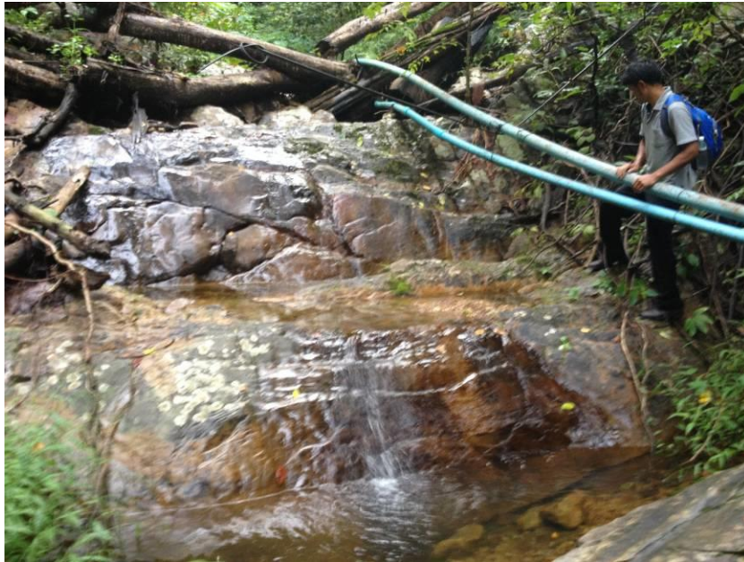
Figure 15: Water distribution system piping in the forest. Water is brought from the source to the 4 major storage tanks near the road. Pipes are above ground due to the rocky landscape.
